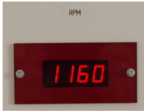
Engine speed control adjuster and speed indicator
