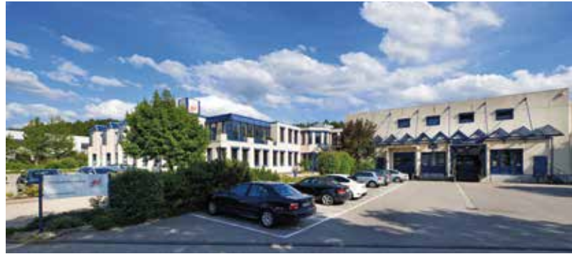
Huf Electronics Bretten, Germany
